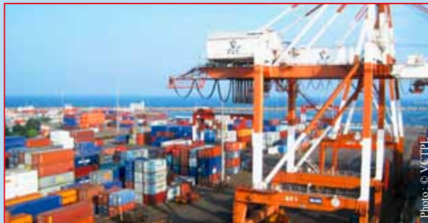
The Visakha Container Terminal at the Port of Visakhapatnam in Andhra Pradesh, India, operates in conformity with the ISO 28000 supply chain security management standard.
